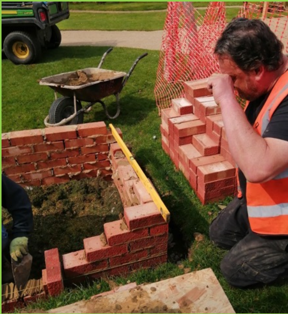
Construction of red brick raised bed to give different colour and texture.
